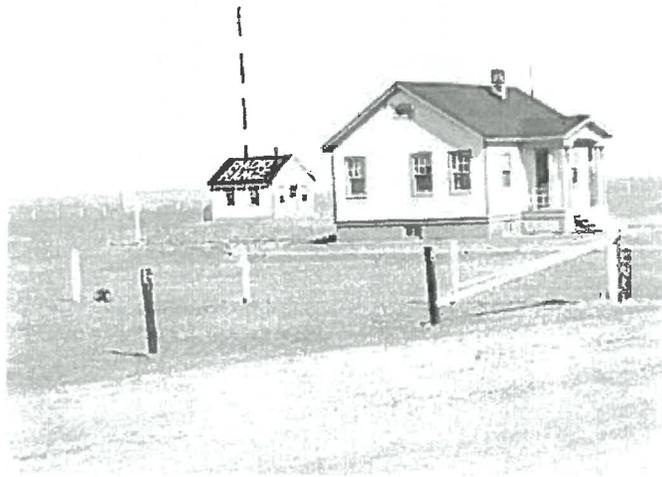
Figure 5. Site 32 Supervisor's house and radio range transmitter building looking northeast (circa 1933). Dimensions of the house were 22 x 28 feet and referred to as "K" quarters. The striped wooden poles, of which there were five, supported the antenna array of the low frequency radio range. Cole-Keller Collection.
