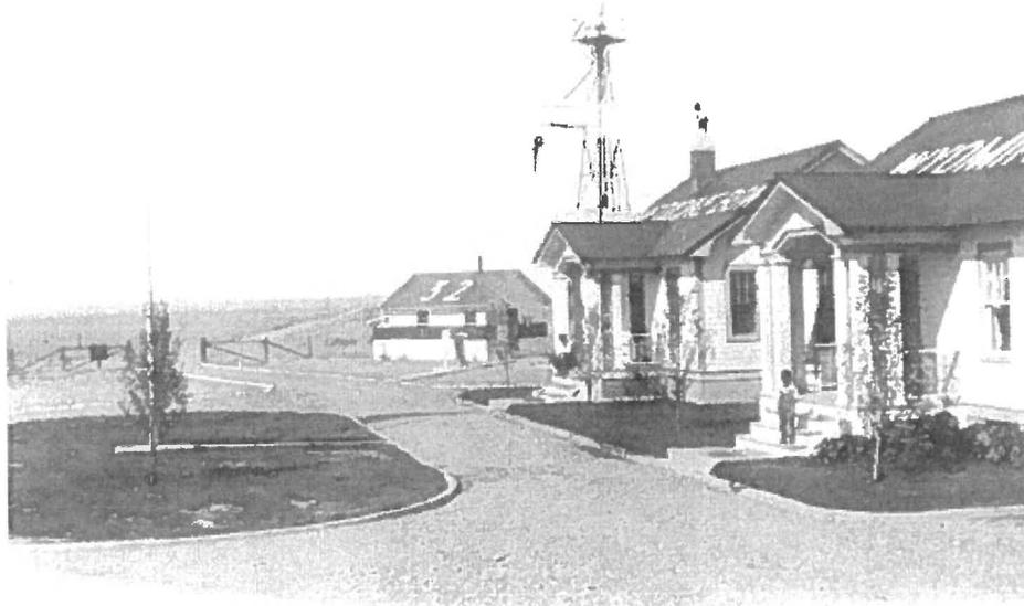
Figure 8. Site 32 office, tower, Airway Keeper's quarters, and flag pole looking northwest (circa 1933) Note well kept grounds and roof lettering to identify the site to pilots. Airway patrol pilots would often note the condition of the site in addition to the operation of the beacon and radio range and report such things as unmown lawns and weeds against buildings to district headquarters.
